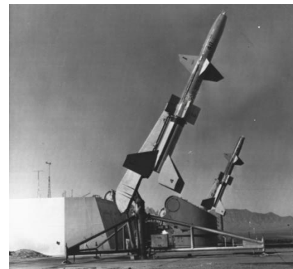
A pair of Talos missiles mounted on USS Desert Ship and being tested for adoption by the U.S. Army. Photo dated October 15, 1957. Talos was a large surface-to-air missile that was mounted on cruisers.
