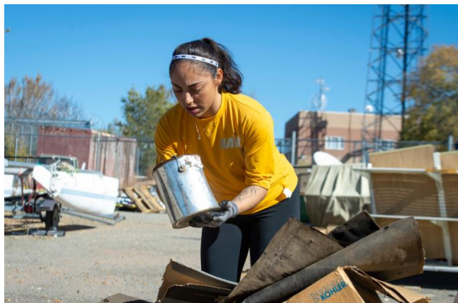
Gunners Mate 3 rd Class Sarah Frank, USS Constitution works on Habitat for Humanity home in Santa Fe
